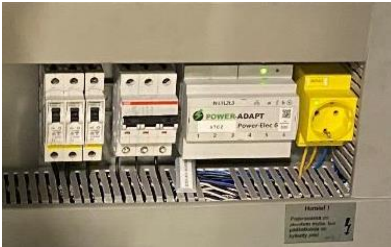
Figure 1: Installation of the measuring unit in a control cabinet (Schaeffler open source)
